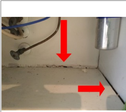
Caulk cabinet under sink
