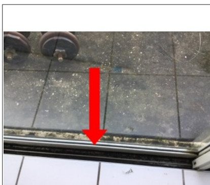
Clean sill plates as derbies is causing resistance as you go to open the sliding glass door.
